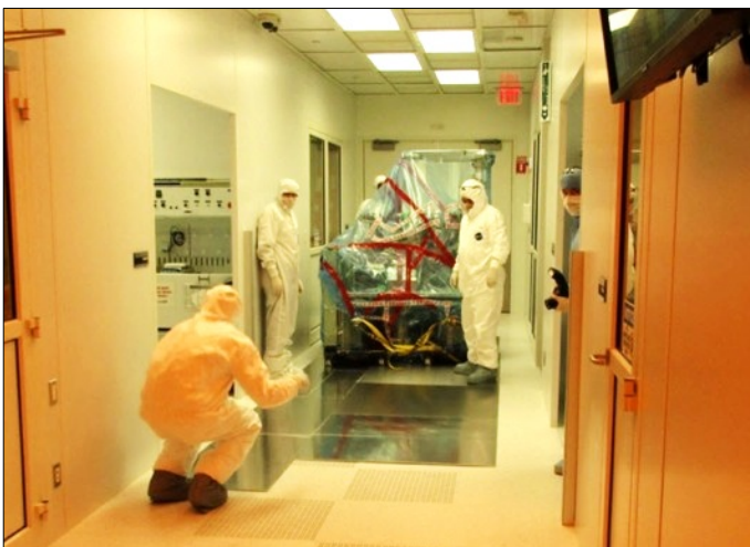
Figure 3: 6300 lb JEOL main console being moved into cleanroom
